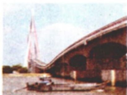
e. Can Tho Bridge
