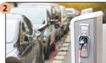
2 add electric charging
